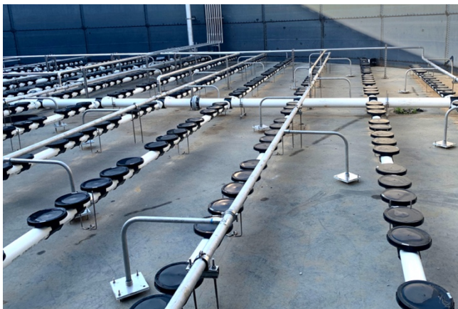
The fine bubble aeration system provides process oxygen while BioMix provides independent mixing.
