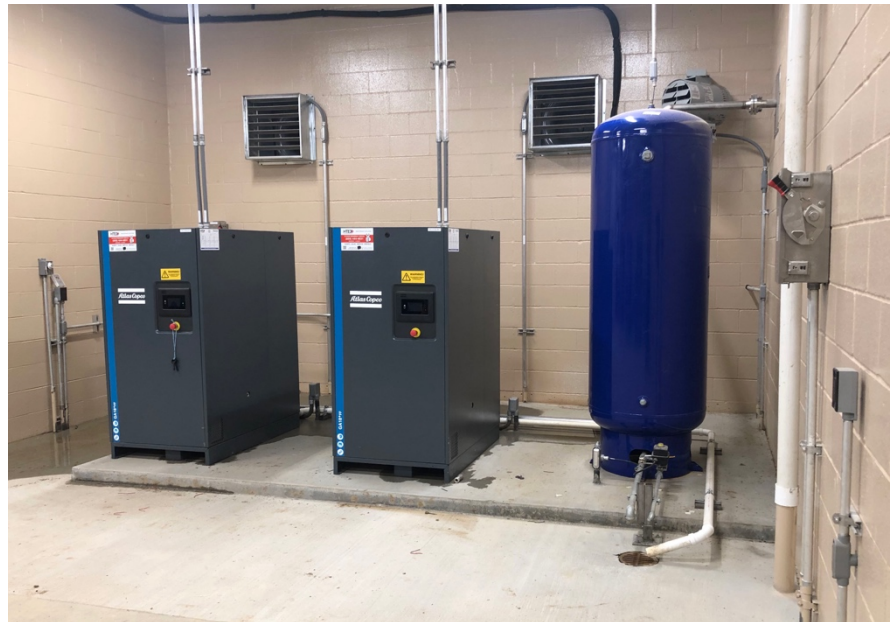
Rotary screw compressors provide high pressure mixing air to the BioMix system.
