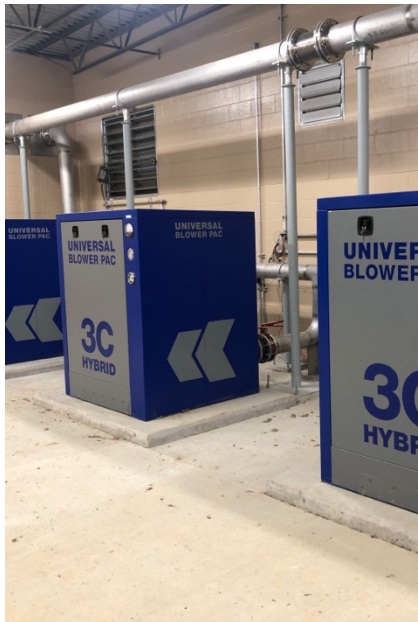
Hybrid blowers provide air to the fine bubble aeration system.
