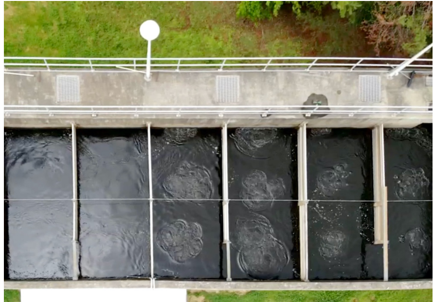
The serpentine flow pattern of the PAC contactor would have required eight mechanical mixers versus two scroll compressors (one duty, one standby)
