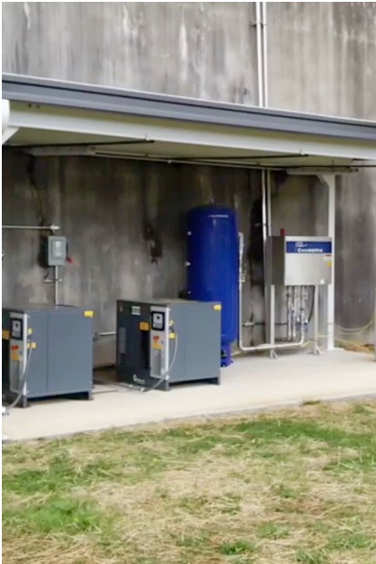
The Zombie valve control module optimally controls mixing regime through operator adjustable settings for duration and frequency of nozzle firing
