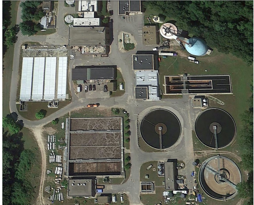
Nashua Wastewater Treatment Facility
