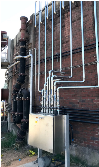
Valve Modules control the firing of compressed digester gas to uniformly mix the digester.
