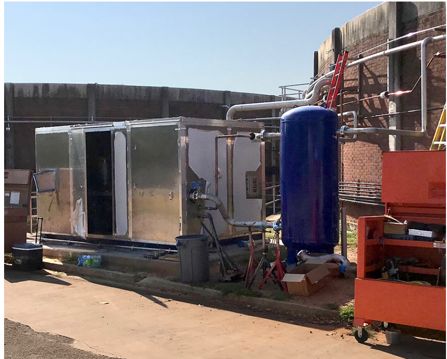
Variable speed duplex biogas compressor package matches system demand.
