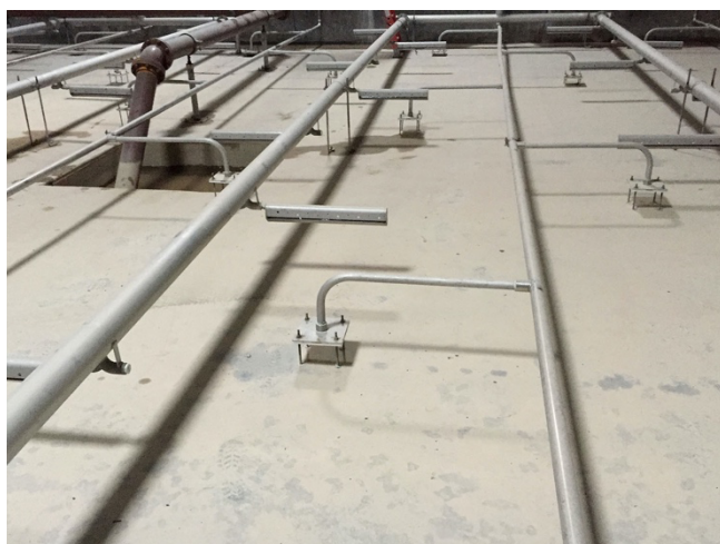
BioMix Compressed Gas Mixing nozzle headers integrated with coarse bubble aeration system
