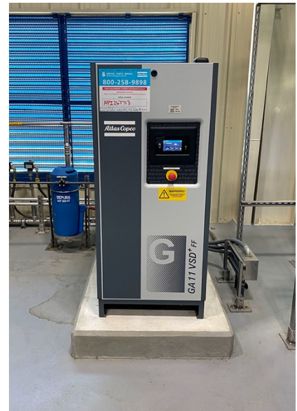
Duty and standby compressors charge the receiver tank which supplies compressed air to the valve module.
