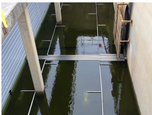
BioMix Compressed Gas Mixing optimizes the anaerobic fermentation process.
