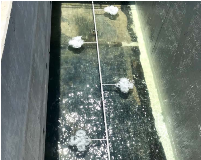
Anaerobic selector basin with BioMix nozzle header firing
