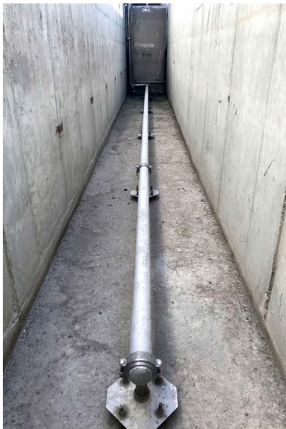
Linear, low profile nozzle header in the anaerobic influent channel
