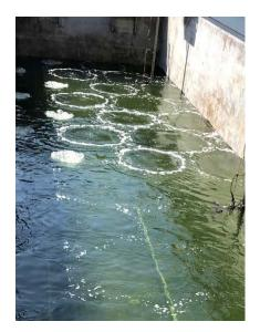
Installing the correct nozzle density is critical in the design of a compressed gas mixing system. Even with a partially full tank, an overlap in the zone of influence of each nozzle can be observed in the surface mixing pattern.
