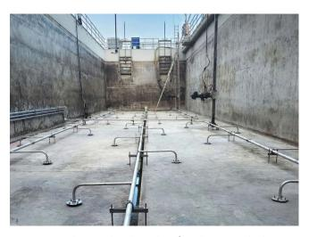
BioMix nozzles are distributed uniformly across the basin floor to provide distributed mixing energy that not only improves efficiency but also prevents solids from settling in the corners of the basins.
