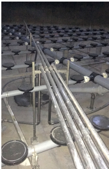
Headers and nozzles easily integrate with the aeration grid and conform to the steep slope of the tank's cone-shaped floor.
