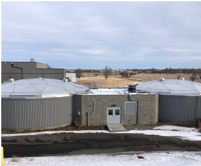
Detroit Lakes WRF's aerobic digesters
