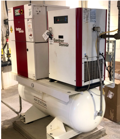
BioCycle-D utilizes compressors to mix the digesters with less than 15% of the horsepower required by the conventional aerated mixing approach.
