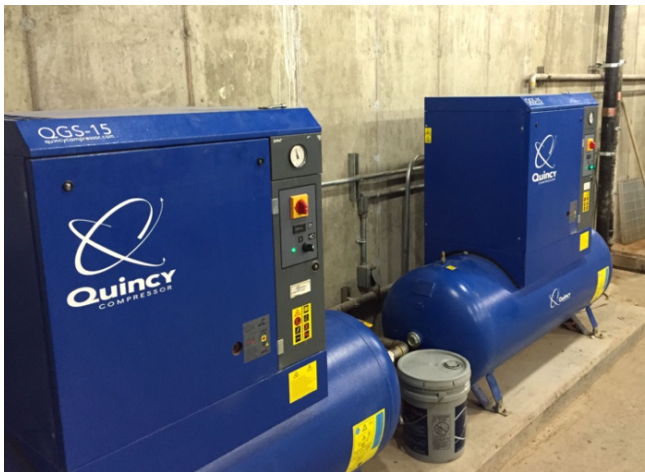
Efficient rotary screw compressors were utilized instead of dozens of submersible mixers.
