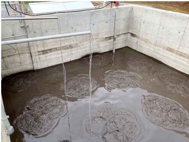
During the anoxic cycle, the BioMix system provides energy efficient and uniform mixing of the sludge.
