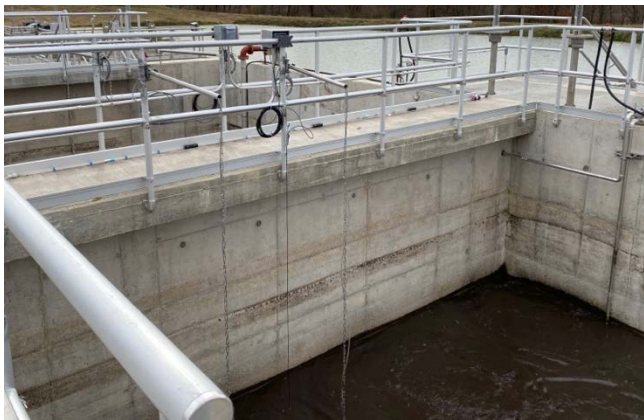
DO and ORP probes provide process feedback to control aerobic and anoxic cycle times.
