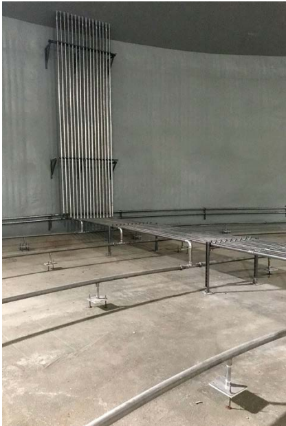
BioMix nozzle headers are designed for any tank geometry or configuration.
