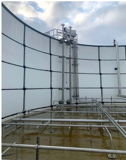
50’ diameter bolt steel tank aerobic digester
