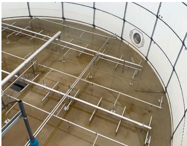
BioMix nozzle headers easily interlace with the coarse bubble aeration grid
