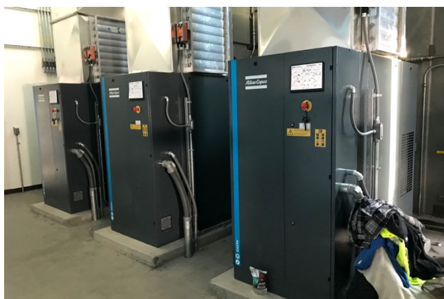
The centralized compressed air system adjusts output to meet the BioMix air demand for mixing multiple applications.
