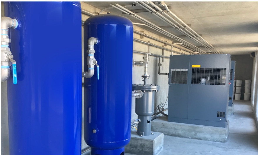
The duty and standby compressors, which are easy to access, are the only components that require routine, scheduled maintenance.
