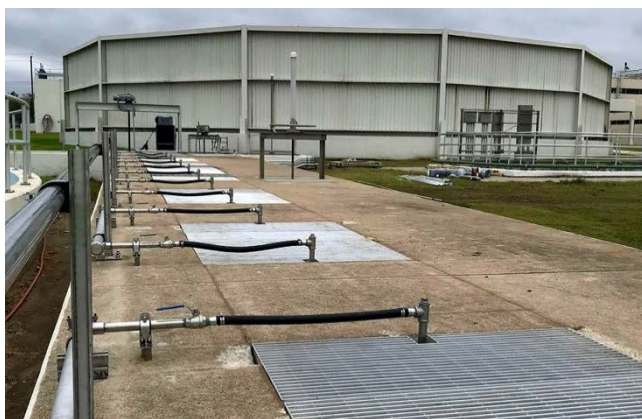
Single drop style nozzle headers uniformly mix the RAS channel
