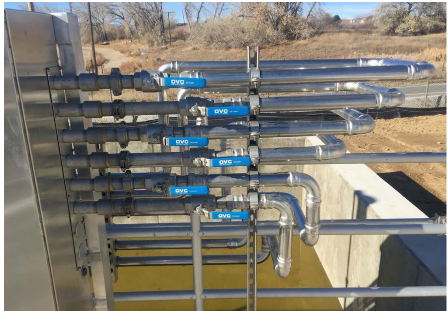
Easy to install press technology piping feeds air to the in-basin nozzle headers
