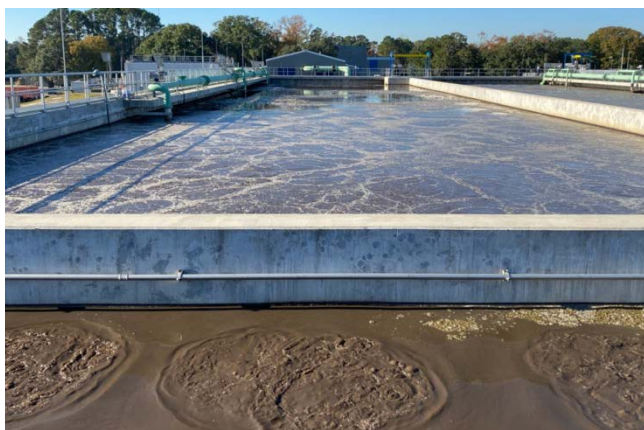
The anoxic zone, mixed by BioMix, provides the optimal conditions for denitrification.
