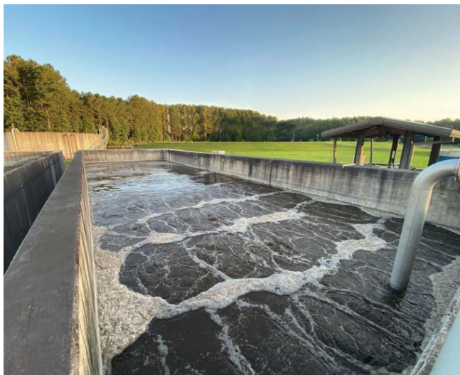
The CAMix system in operation at the Cherry Point WRF
