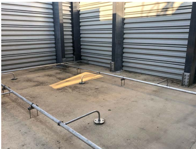
BioMix nozzle headers installed on the tank floor of an anoxic selector in Phase I.
