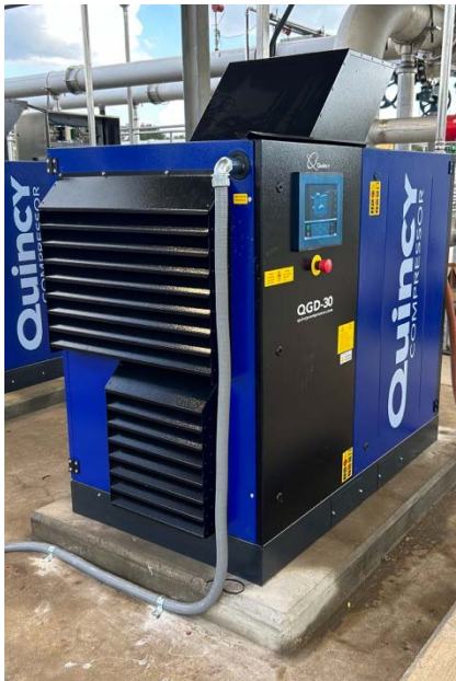
Duty and standby rotary screw compressors serve the BioMix system.
