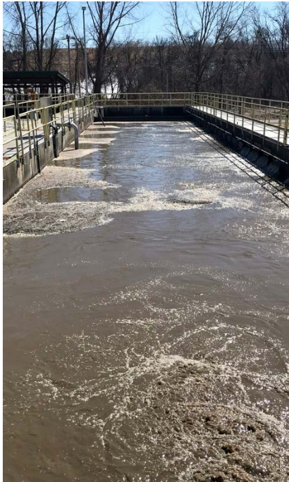
BioMix provides complete mixing with negligible oxygen transfer.
