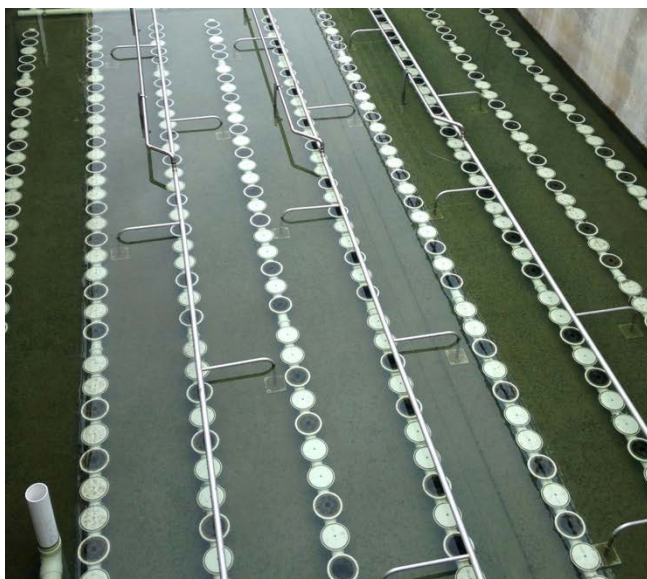
BioMix nozzles and headers easily integrate with aeration equipment in the anoxic zones.
