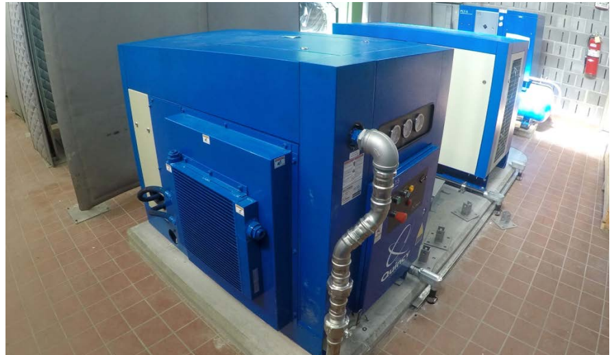
BioMix is powered by a duty and standby compressor system housed in a controlled environment.
