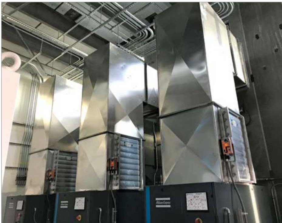
Exhaust ducts solve the issue of heat rejection at a facility in Olympia, WA.
