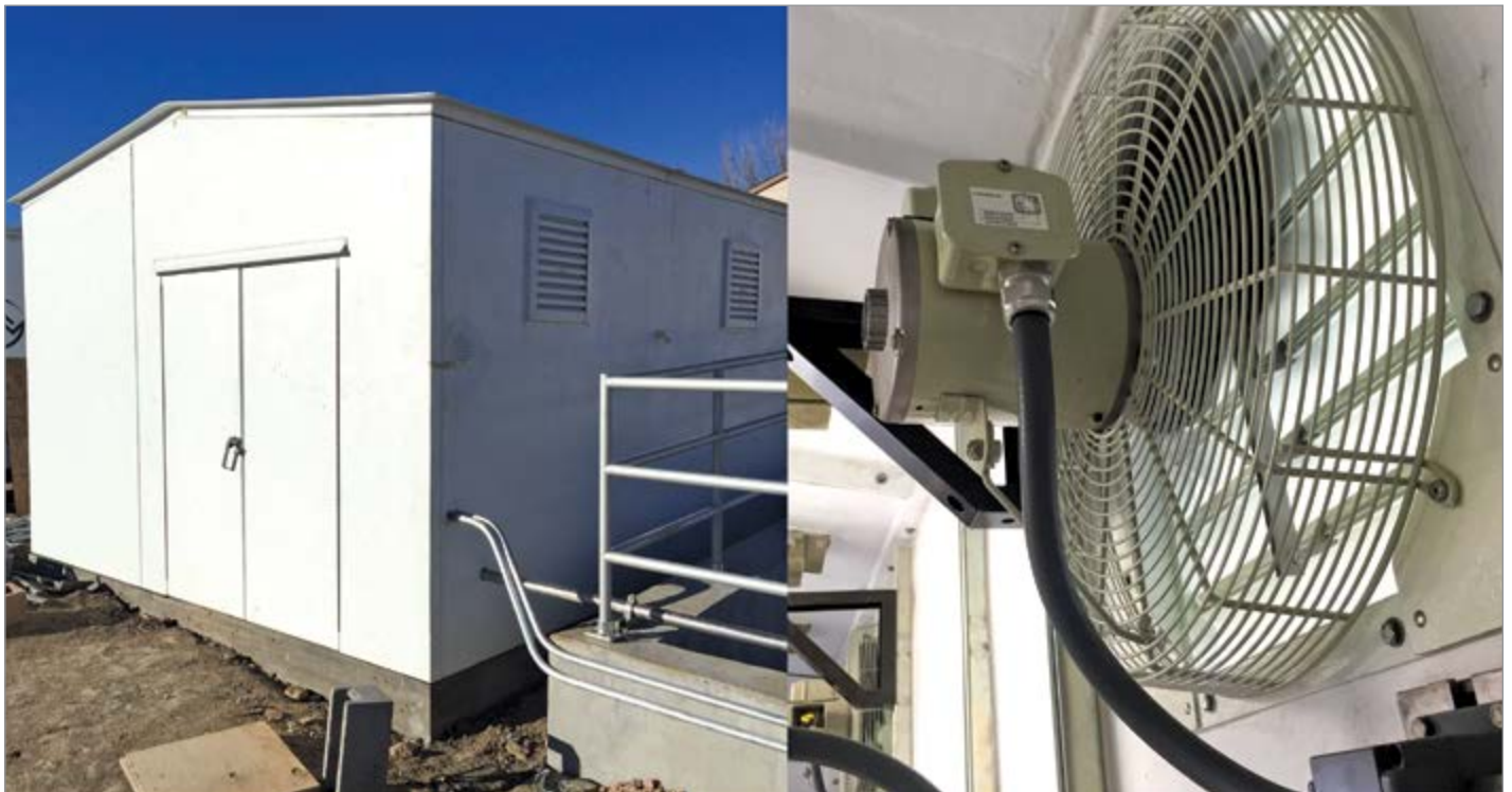
Two exhaust fans are incorporated into an environmental enclosure at a facility in Widefield, CO
