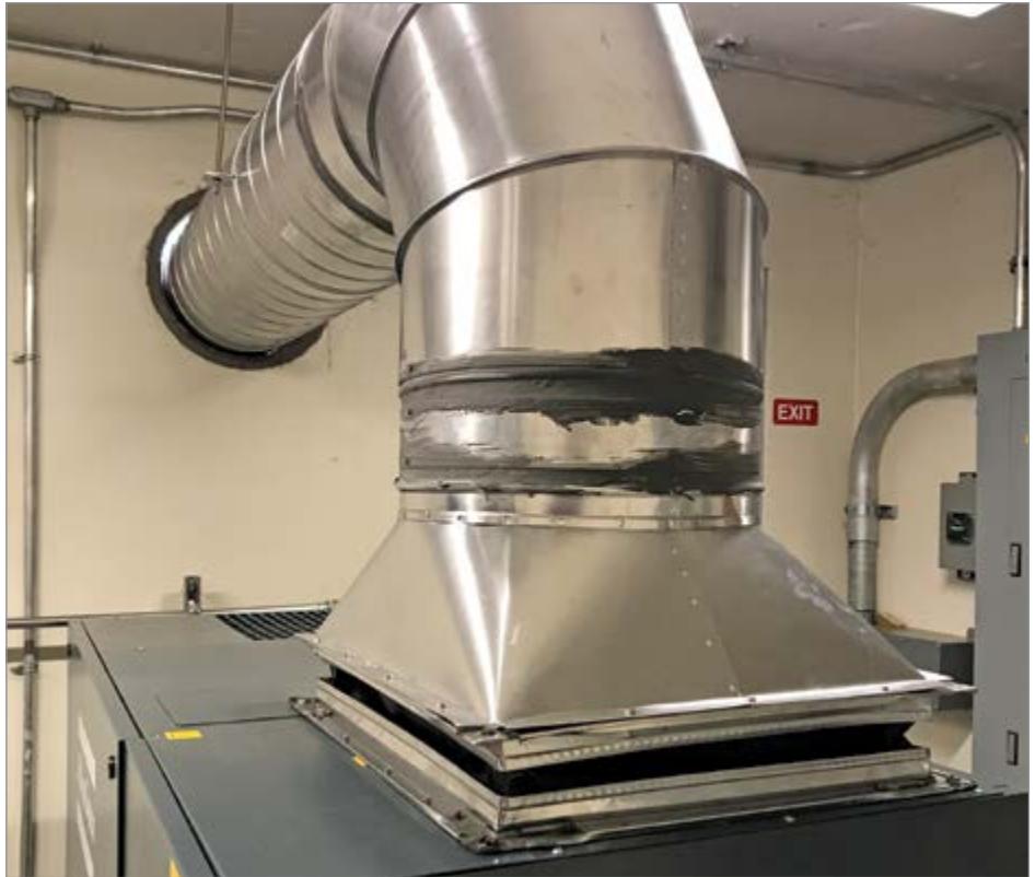
Heat is conveyed out of the air compressor room by an exhaust duct at a facility in Somersworth, NH.
