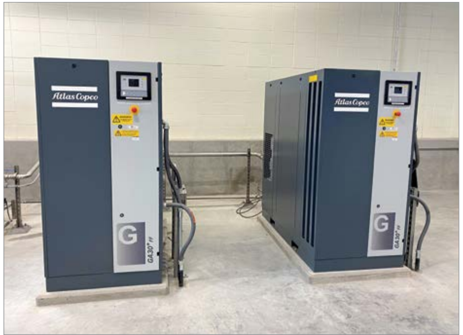
Indoor duty and standby air compressors at a facility in Castle Rock, CO
