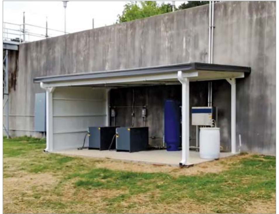
This air compressor, receiver tank and valve module are housed under a tankside canopy in Monroe, NC.
