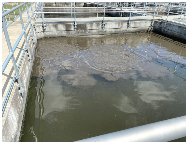
SGWASA’s Anaerobic Selector
