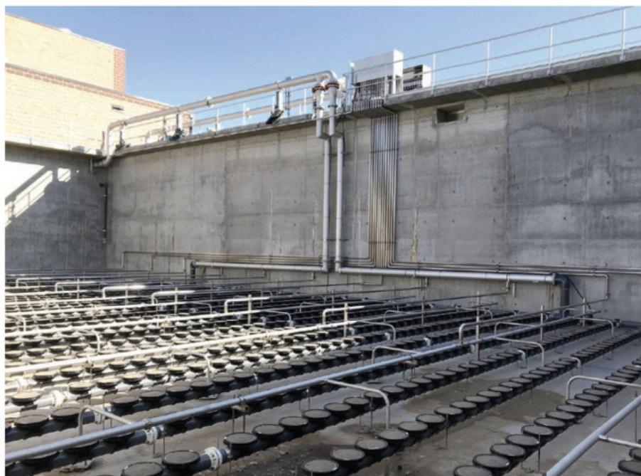
Compressed gas mixing nozzles integrate easily with aeration equipment.
