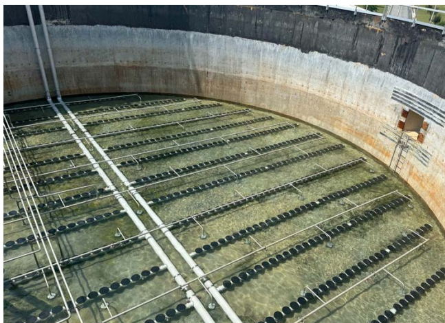
De-coupling aeration from mixing optimizes efficiency and process control.
