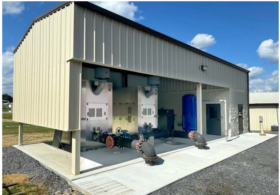
The blowers, compressor system, and receiver tank for the aerobic digesters are easily accessible and protected under a canopy.
