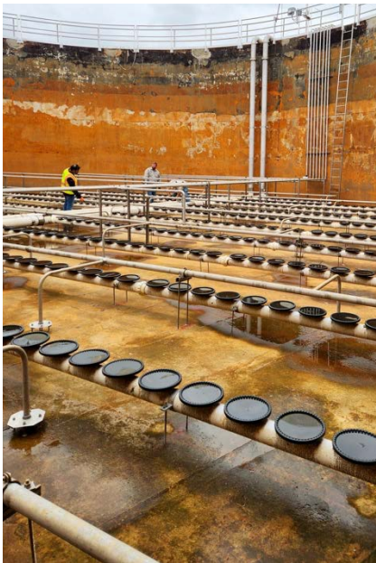
Compressed gas mixing nozzles are interlaced with aeration equipment.
