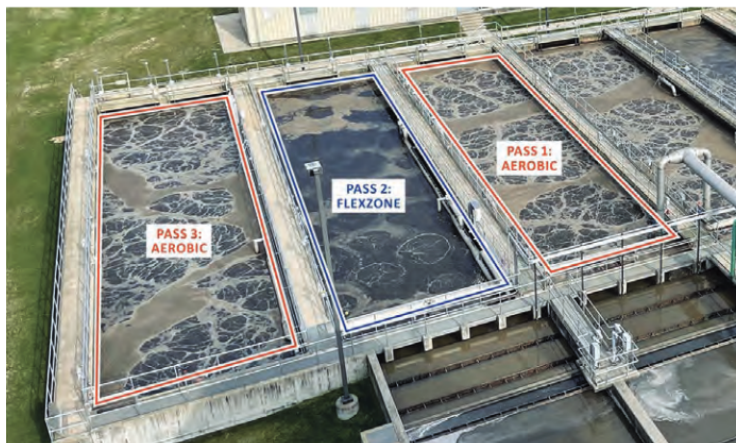
The FlexZone process is installed on the second pass of each three-pass aeration train at the Grandville plant. The first and third passes remain aeration only.
